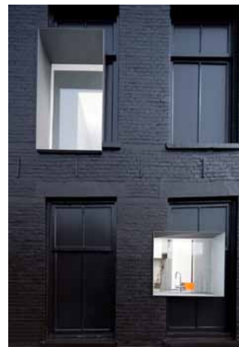
THE OLD WINDOWS HAVE BEEN CLOSED UP AND PAINTED BLACK. NEW WINDOWS POKE THROUGH THE FAÇADE IN A STEEL CASING.
