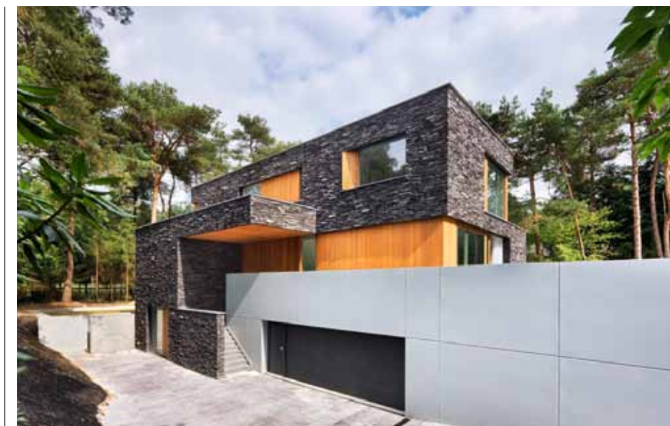
A LONG CONCRETE RETAINING WALL DIVIDES THE GROUND FLOOR FROM THE SLOPING RAMP DOWN TO THE SUNKEN GARAGE.
