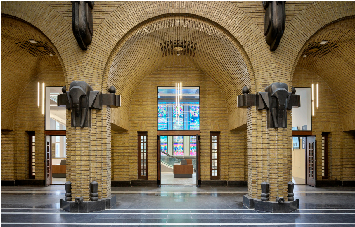
Openings created above the characteristic historical doors provide light and new sight lines.
